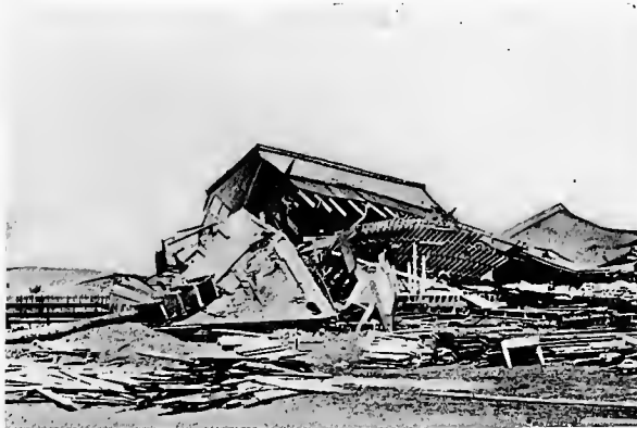
E. Haywards. Wreck of buildings by earthquake of 1868.
